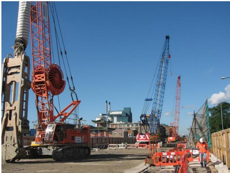
*Rigs operating over the working platform stabilised with Tensar TriAx<sup>®</sup> geogrids*
