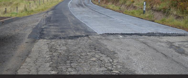
Tensar AX5-GN asphalt interlayer installed onto a 20mm regulating layer.
