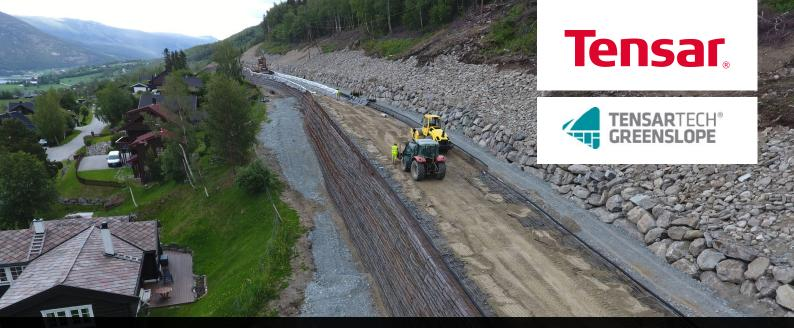
Tensar's GreenSlope reinforced earth slope system delivered a cost-effective alternative for constructing the rockfall protection bund, using locally-sourced fill.
