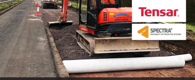
A Tensar geocomposite of stabilisation geogrid backed with a non-woven geotextile was laid in a single layer, stabilising the road's sub-base and offering resistance to upwards migration of fines due to groundwater conditions
