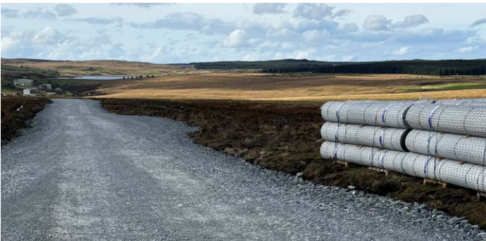
Stranoch Onshore Wind Farm
