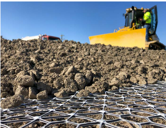
Granular particles interlocking with the Tensar InterAx structure.
